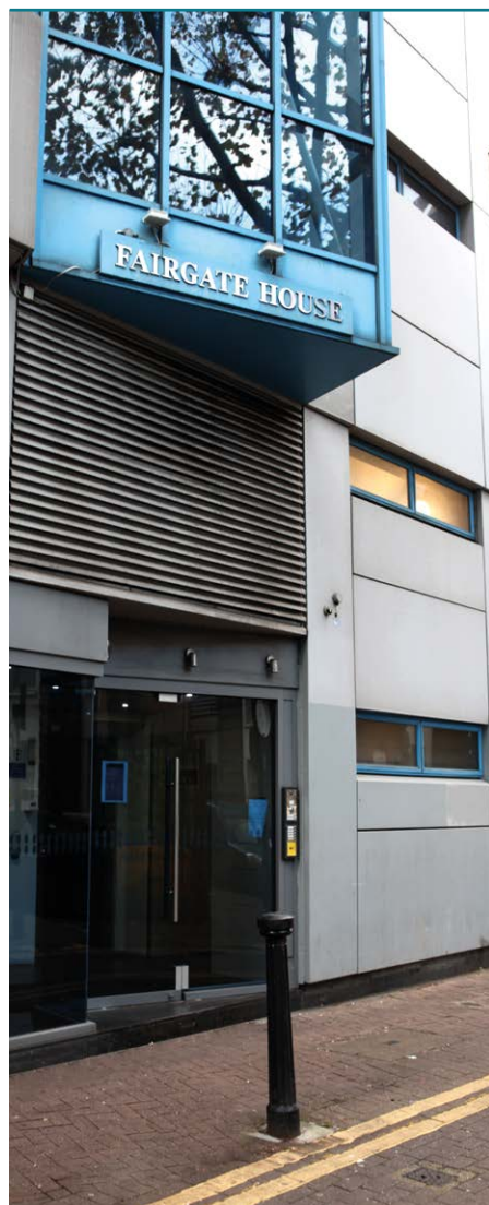
SH Landes' former office was in this building just off New Oxford Street in London
